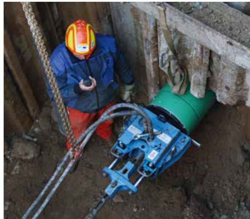
Picture left: the new PP pipes ND 450 had to be handled by crane • Picture center: Crews in the machine and reception pit keep constant radio contact while the new PP pipes are being pulled in. Picture right: The bursting head with new pipe attached has arrived in the machine pit.
