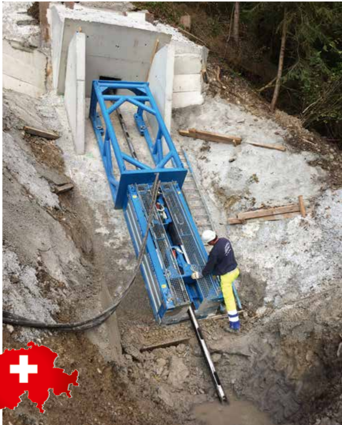
The GRUNDOBURST 19006 with its attachment frame, installed in the work pit.
