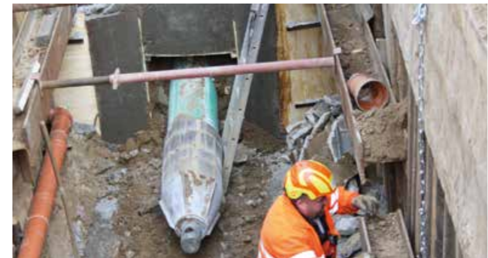
Picture left: the new PP pipes ND 450 had to be handled by crane • Picture center: Crews in the machine and reception pit keep constant radio contact while the new PP pipes are being pulled in. Picture right: The bursting head with new pipe attached has arrived in the machine pit.
