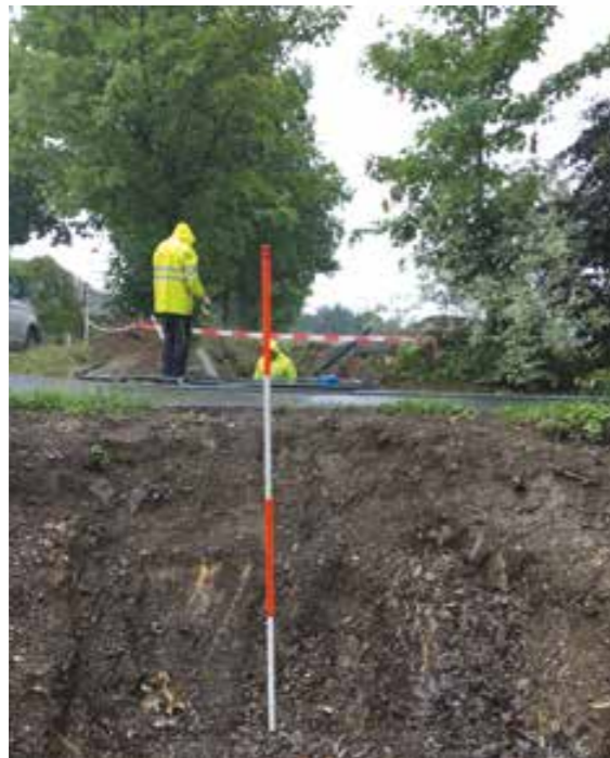
View from start to exit pit.
