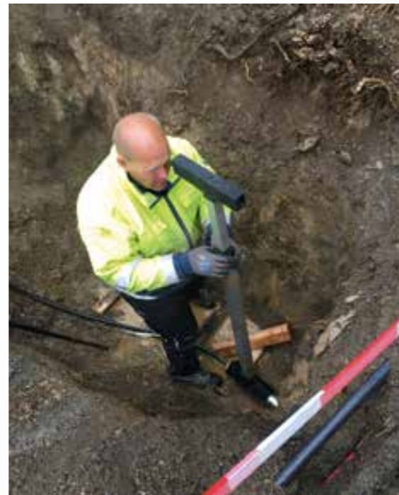
The installation required utmost precision.
