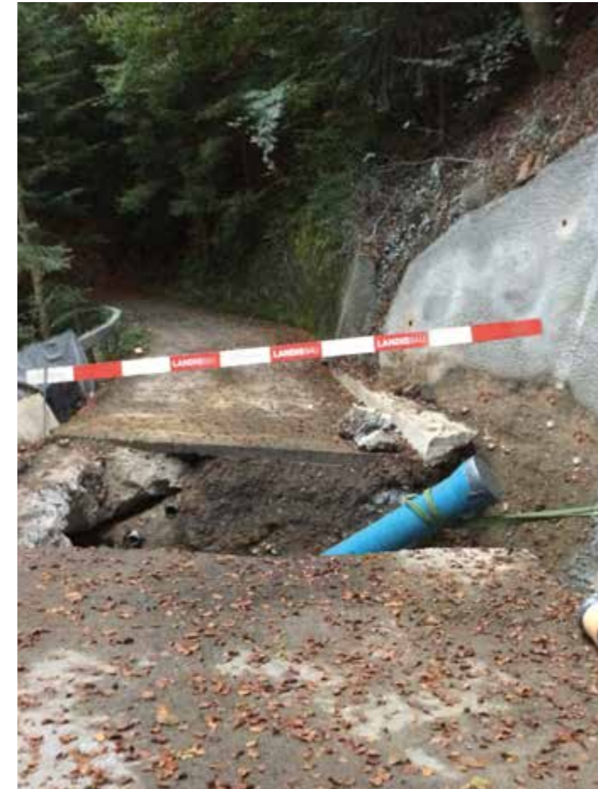
The smaller PE-coated ductile cast iron pipe ND 250 after installation.
