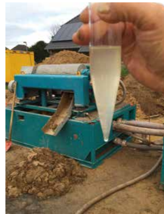
Picture left and centre: The new SRU2017 trailer. Deployed for the company REVOR to create a complicated 400 m long rock bore in Lohmar.
