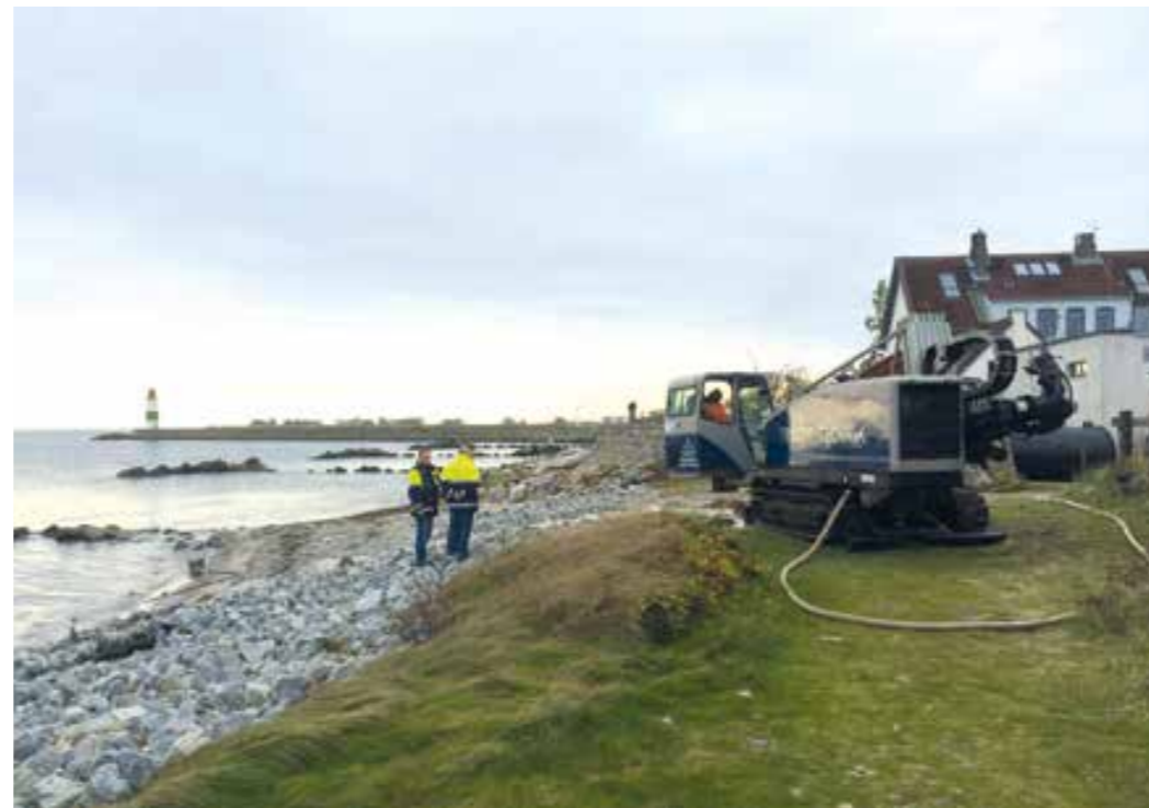
The restored surface on the mole.
