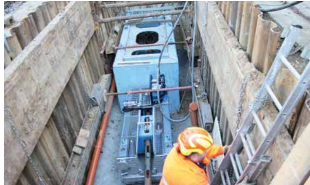
Picture left: The bursting head • Picture center: GRUNDOBURST 2500G with support from inside the construction pit. • Picture right: The Quick-Lock bursting rods.
