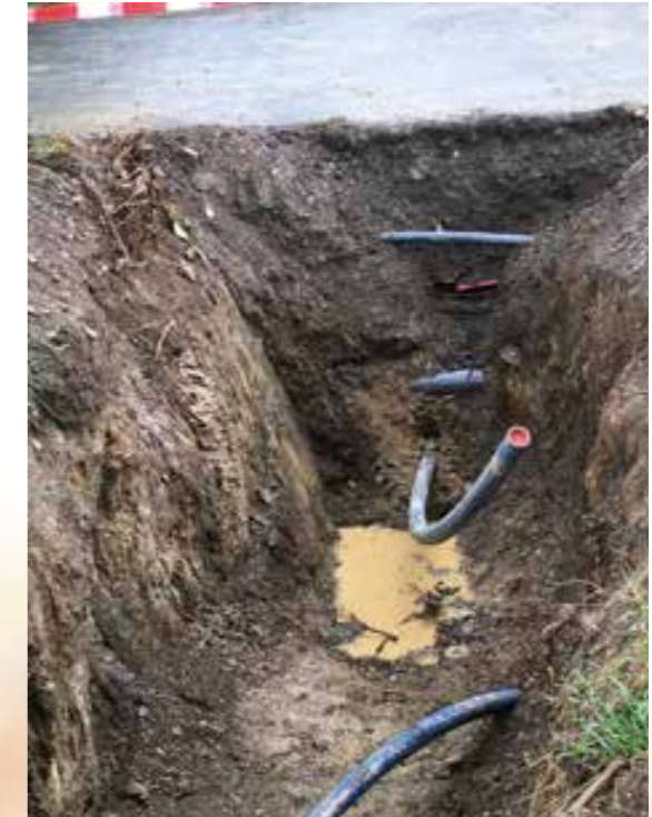
The new water line.
