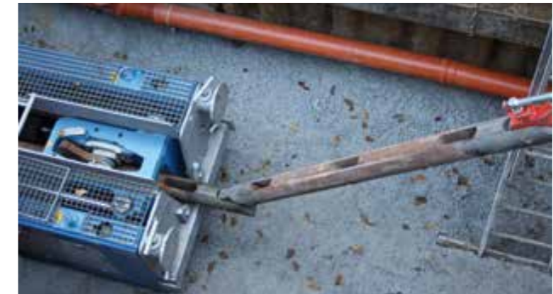
Picture left: The bursting head • Picture center: GRUNDOBURST 2500G with support from inside the construction pit. • Picture right: The Quick-Lock bursting rods.
