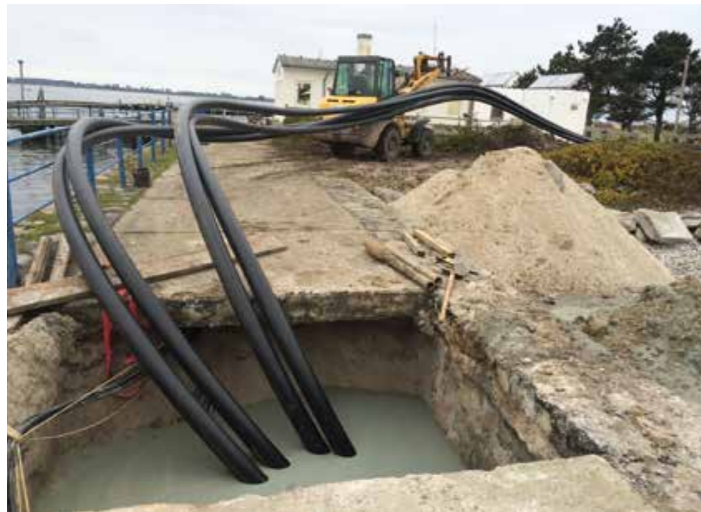
The target pit in the mole while the pipe was pulled in.
