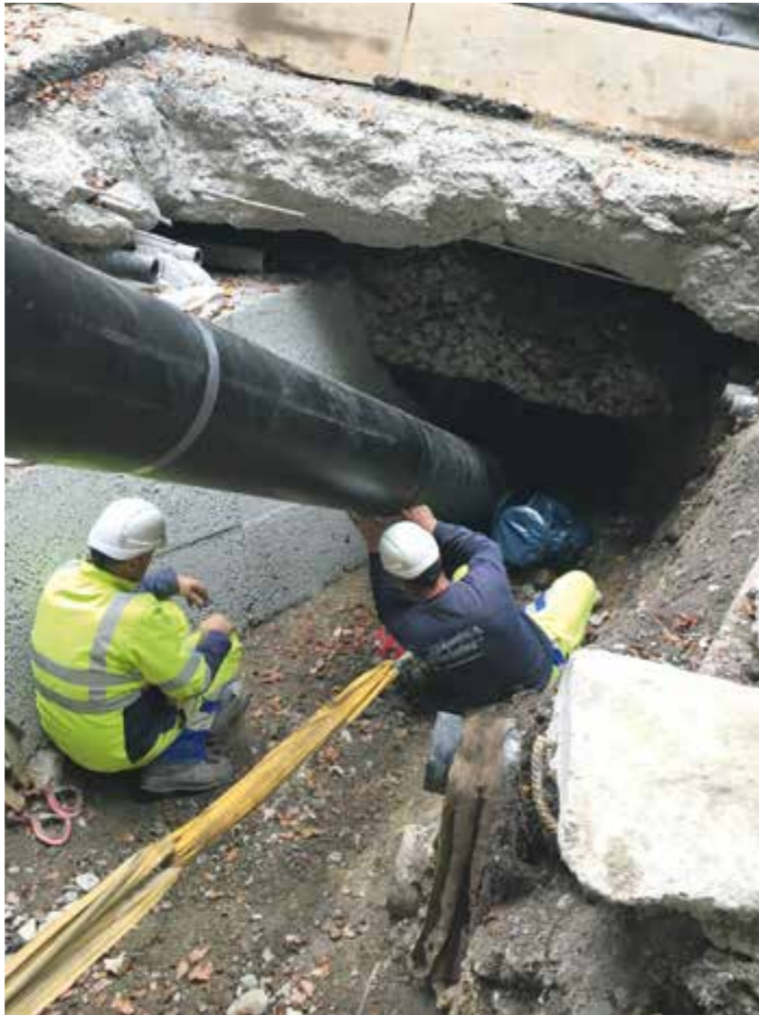
The new PE-coated ductile cast iron pipe ND 300 in the process of installation.
