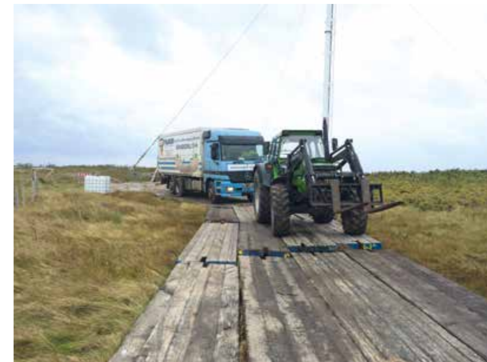
With tractor support: transporting the drill truck through the protected landscape.
