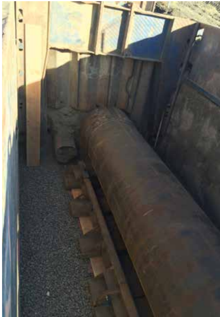
Crews rammed Ø 1.200 mm steel casings at the launch and exit pits to seal off and prevent ground water from entering during drilling operations.
